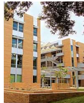
UCR Engineering Building
