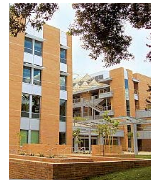
UCR Engineering Building
